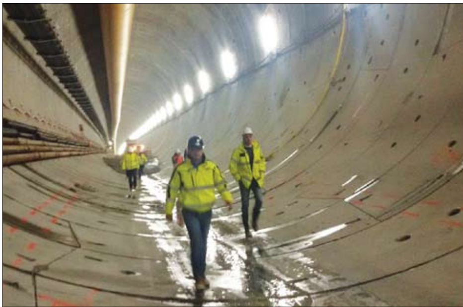
SS 640 Porto Empedocle – Galleria Caltanissetta- Italia
