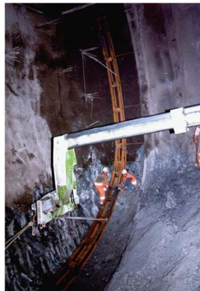
Figure 9 Detail of the strut in the tunnel invert
