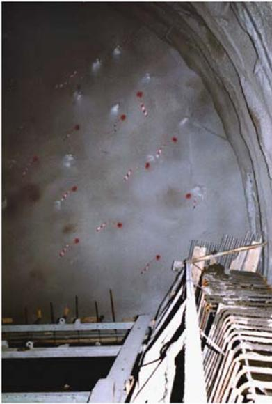
Figure 3 Detail of the positioner during the installation of fibre glass elements
