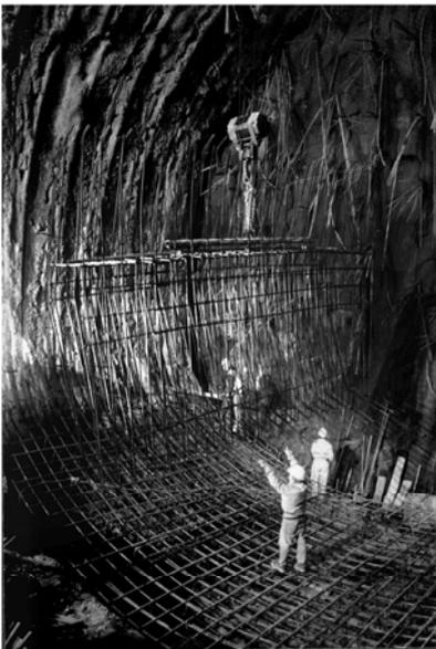
Figure 11 Placing reinforcement for the tunnel invert
