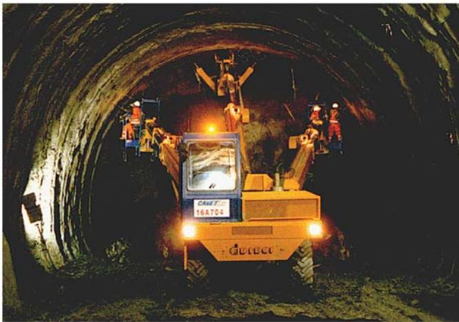
Figure 8 Placing the preliminary lining
