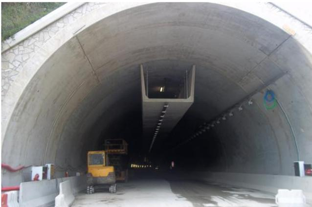
Figure 16. Sellero tunnel – Detail of the prefabricated structure
