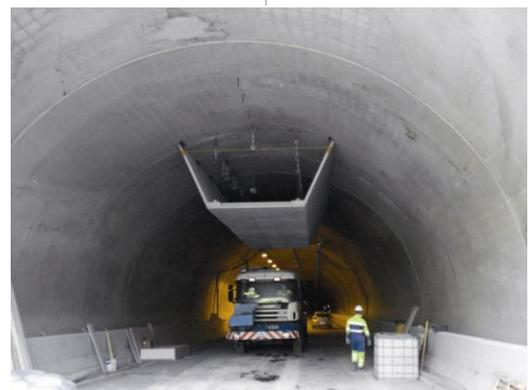
Figure 3. Suspended Escape route within the cross section of Macina tunnel (Carrara)
