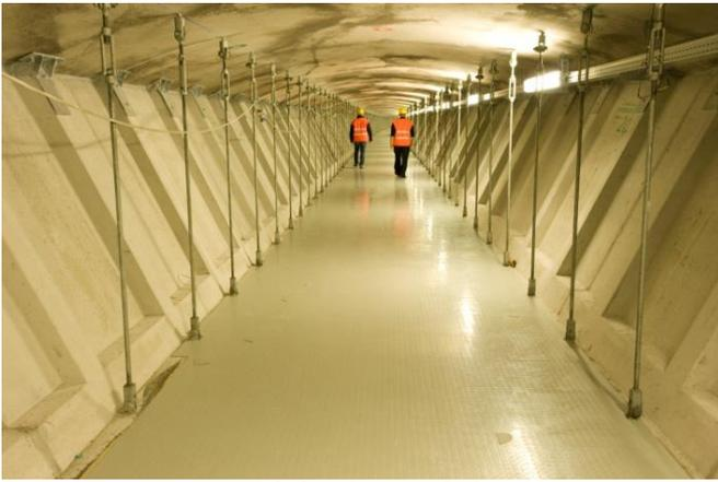
Figure 4. Interior of the Suspended Emergency Escape Route
