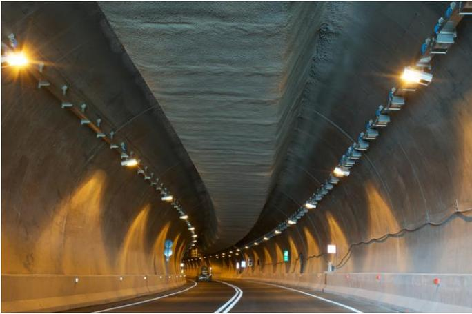
Figure 15. Macina tunnel- Completed Suspended Emergency Escape Route
