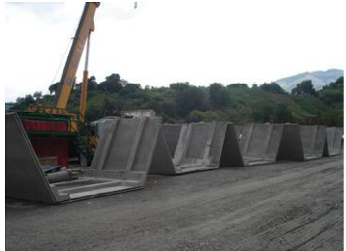
Figure 7. Precast segments of Suspended Escape Route stored on site (Macina and Monte Greco tunnel, Carrara)
